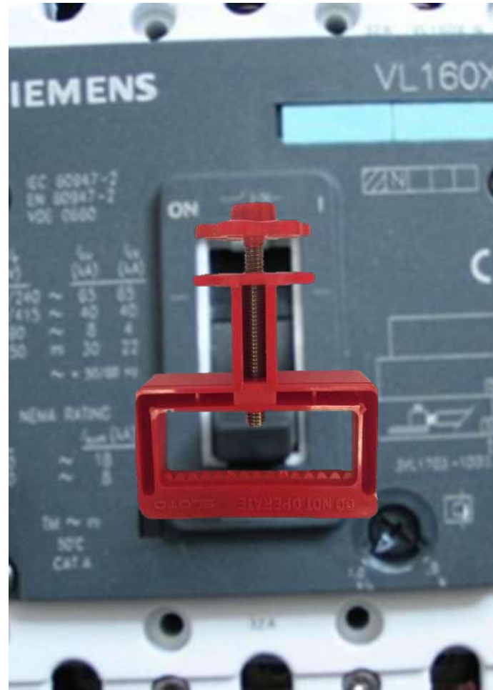
MCCB Lockout (Screw type)
