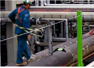
Pipe Rack Lifeline System
